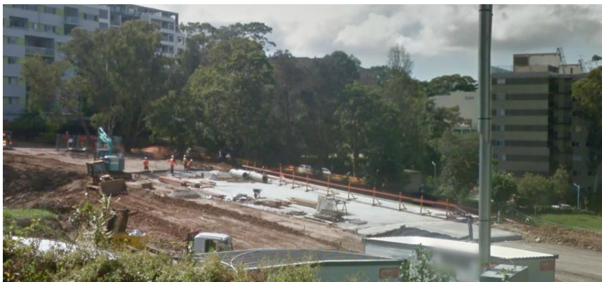
Figure 5: Construction of Waterview Drive (image: Google Maps, April 2014)
